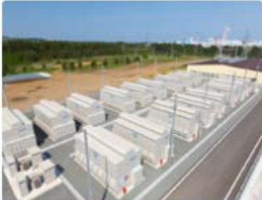
NGK 34 MW NAS alongside 51 MW Wind Farm
